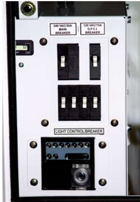
Engine control panel hour meter, breakers, light switches and key start
